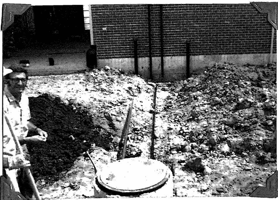
TANK INSTALLATIONS FOR DIESEL FUEL, HEATING FUEL + WASTE OIL ON WEST SIDE OF NEW ADDITION TO SERVICE EQUIPMENT BUILDING AS IT WAS NEARING COMPLETION IN JUNE + JULY-1974.
