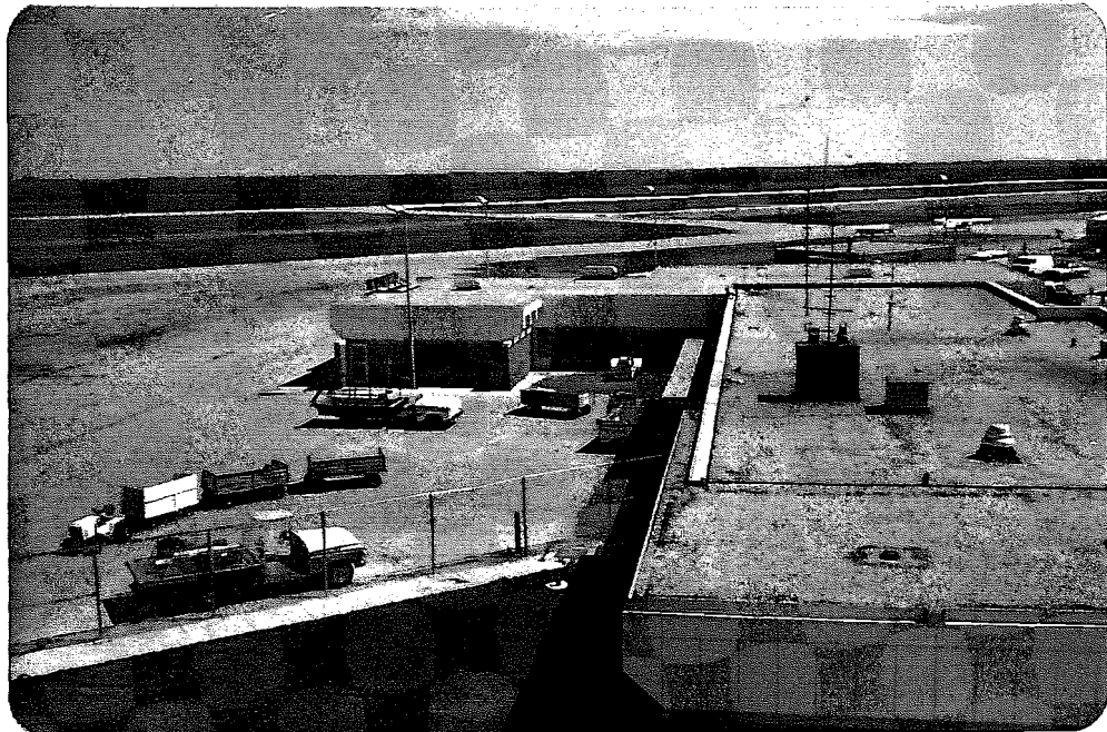
ABOVE PICTURE SHOWS WORK IN PROGRESS IN JUNE-1978 ON EARTH WORK FOR SECOND SEGMENT OF EAST-WEST PARALLEL TAXIWAY. GRAVEL FILL ALSO BEING HAULED IN FOR SUB-BASE IN PREPARATION FOR PAVING.
