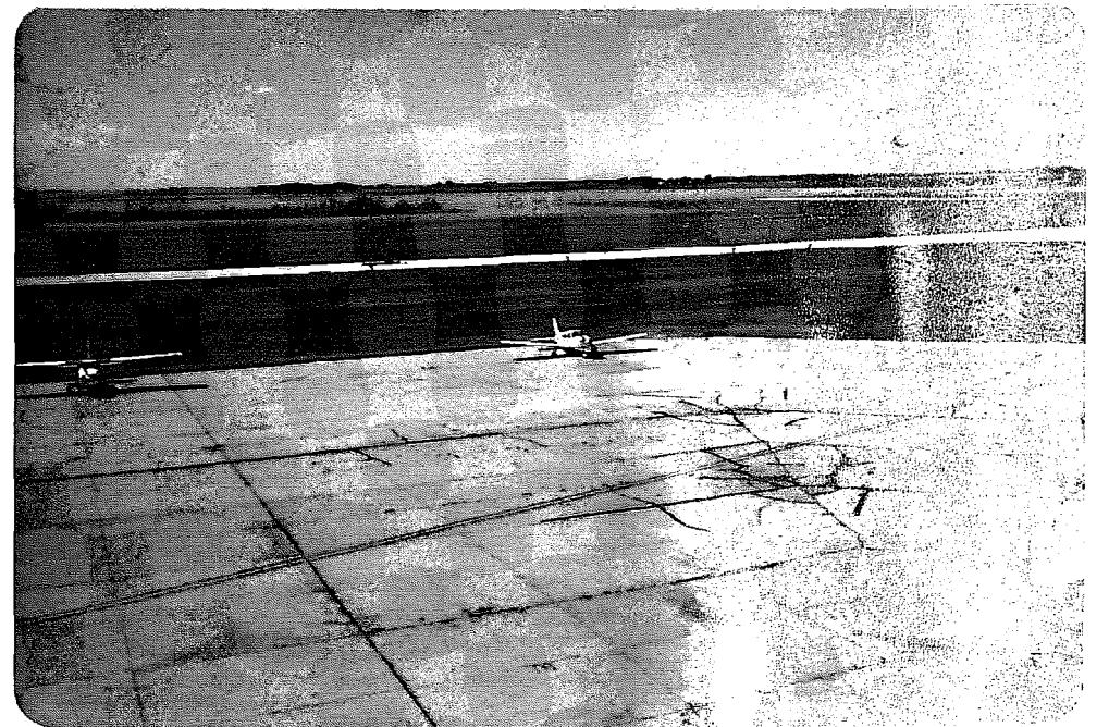
HERE WE SEE THE N-S PARALLEL TAXIWAY PAVING AS IT LOOKED COMPLETED AND ALL THE BLACK DIRT COVER SPREAD OVER SLOPES, EDLING ELECTRIC WORKING ON TAXIWAY EDGE LIGHTING IN LATE JUNE-1978.
