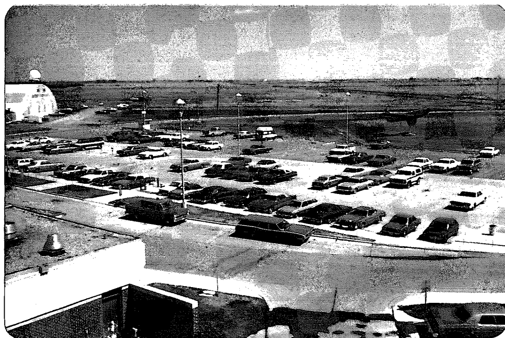
ABOVE PICTURE SHOWS BLACK DIRT COVER AND FINAL GRADING OF N.G. EARTH FILL AREA AFTER CARL PAULSON AND AIRPORT CREW COMPLETED PROJECT, JULY-1978
