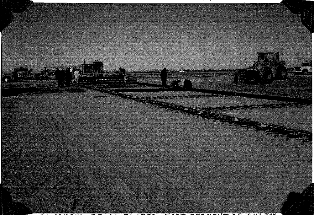
CONCRETE BEING POURED - EAST SEGMENT OF EW TAX.
