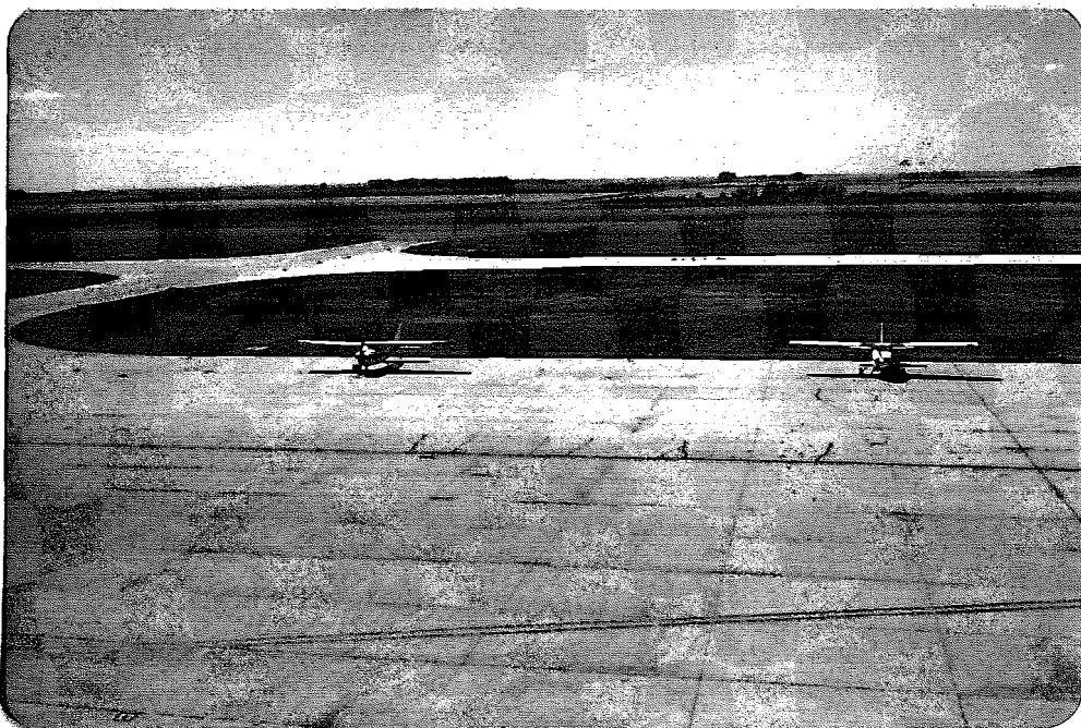
HERE WE SEE THE N-S PARALLEL TAXIWAY PAVING AS IT LOOKED COMPLETED AND ALL THE BLACK DIRT COVER SPREAD OVER SLOPES, EDLING ELECTRIC WORKING ON TAXIWAY EDGE LIGHTING IN LATE JUNE-1978.
