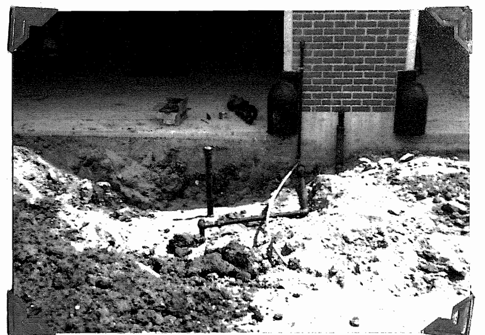
TANK INSTALLATIONS FOR DIESEL FUEL, HEATING FUEL + WASTE OIL ON WEST SIDE OF NEW ADDITION TO SERVICE EQUIPMENT BUILDING AS IT WAS NEARING COMPLETION IN JUNE + JULY-1974.
