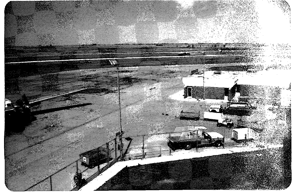
HERE WE SEE COMPLETED PAVING ON SECOND SEGMENT OF E-W PARALLEL TAXIWAY AND BACK FILL OF BLACK DIRT IN PROGRESS IN JULY-1978, 1ST RUN ON CONCRETE WAS POURED JULY 20TH.
