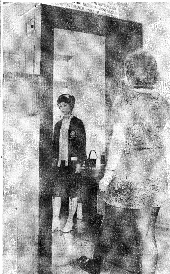
PASSENGERS AT THE Grand Forks International Airport have a new "doorway" to walk through before boarding their airliner. Called a "magnometer," the structure is a metal-detecting device installed to comply with new antihijack measures required by Federal Aviation Authority requirements. It is operated by representatives of the Pinkerton Detective Agency, such as Marie Charette shown in the background. (Herald photo)
