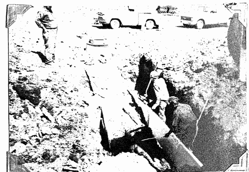
RELOCATION AND REPLACEMENT OF SOME SEWER LINE IN CONNECTION WITH PAVING OF SERVICE ROAD TO U.N.D. FACILITY IN JUNE-1974.
