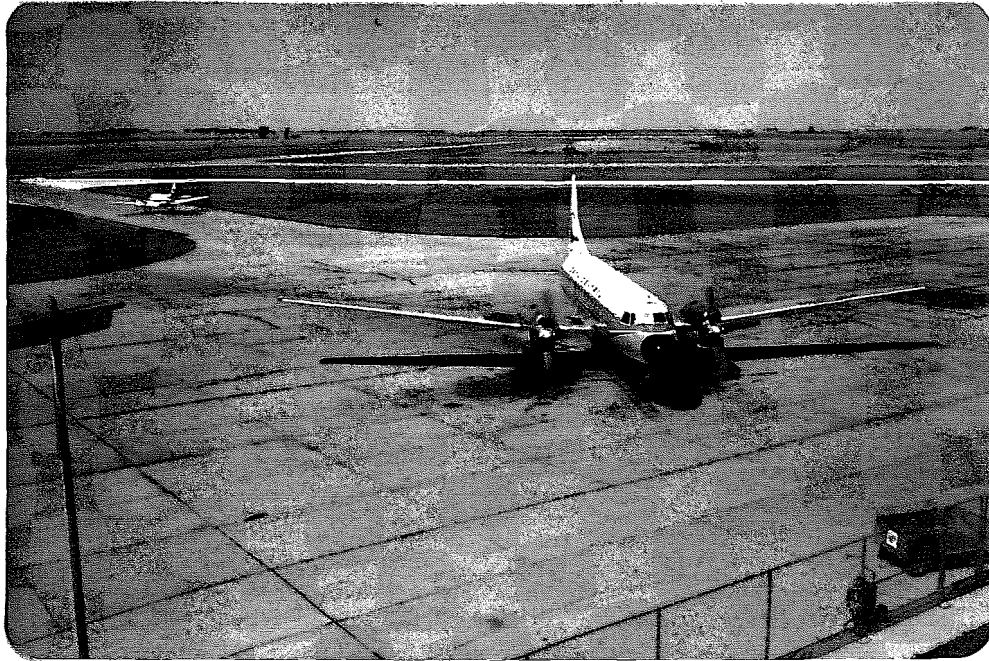
HERE WE SEE COMPLETED PAVING ON SECOND SEGMENT OF E-W PARALLEL TAXIWAY AND BACK FILL OF BLACK DIRT IN PROGRESS IN JULY-1978, 1ST RUN ON CONCRETE WAS POURED JULY 20TH.
