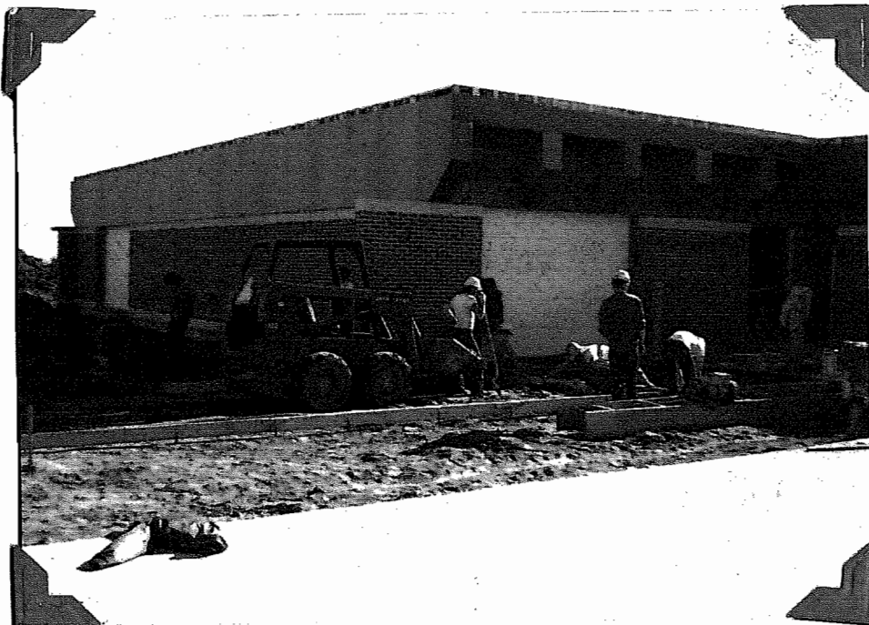
NODDY CONTRACTING BEGINNING TO PREPARE BASE AND POUR CONCRETE SLAB FOR ACCESS TO BAGGAGE PICKUP AREA, SEPTEMBER 1974
