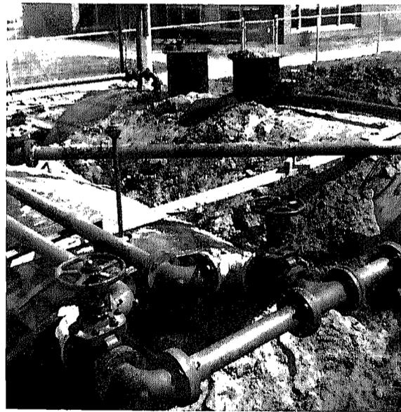
JET FUEL TANKS BURIED SHOWING PLUMBING INSTALLED IN MAY-1967
